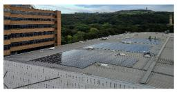
Despite the challenge to complete works during the COVID shutdowns, Estates & Facilities took the opportunity to undertake construction and improvement works including installing 422 Solar Photovoltaic panels on Technology Building which will generate 150,000 kWh of electricity annually.
